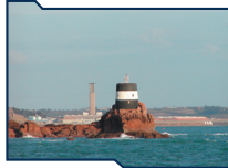
NOIRMONT TOWER (11M)
